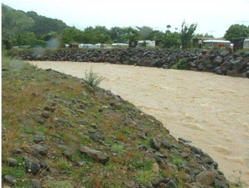
Figure 13 Engineering works undertaken on the Te Puru Stream
